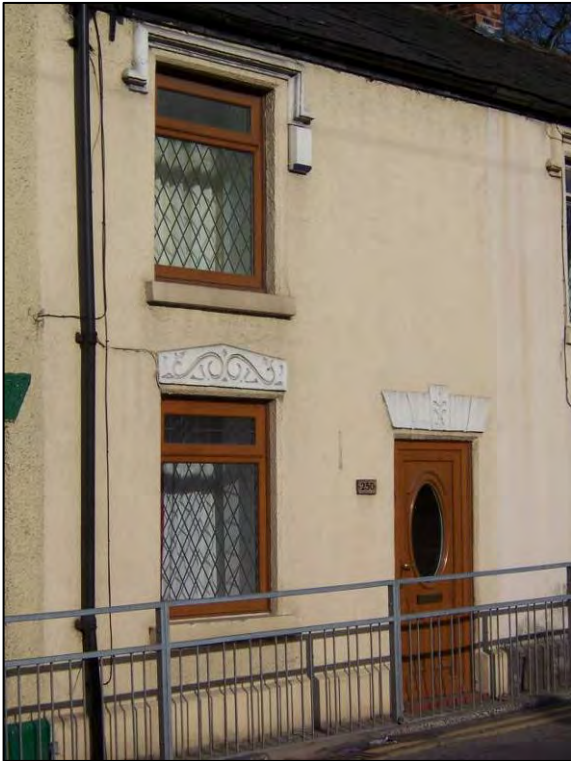
Stone detailing to Andrew Street terraced houses. Upper windows have Tudor-style hood moulds, while ground storey lights have shaped lintels with incised decoration. Door lintels are wedge-shaped and rusticated with incised keystones. These small houses are unusual within the village in being so elaborately decorated.
