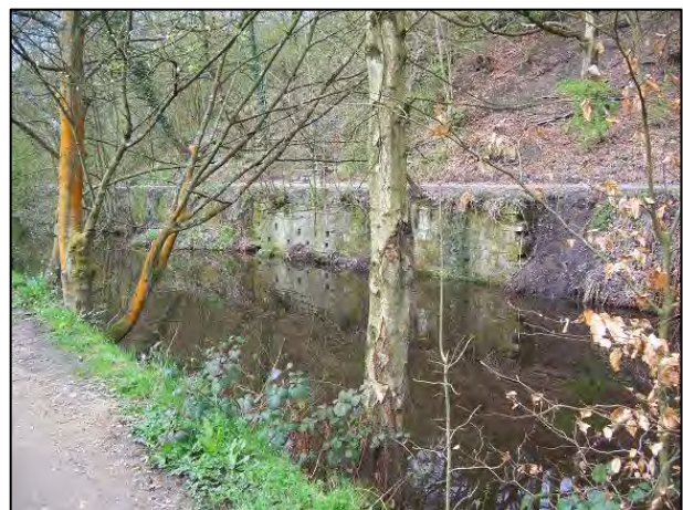
Mill leat, designed as a canal with masonry retaining walls and a quayside for loading coal from the tramway to barges.
