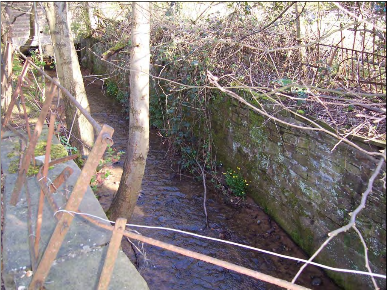
Culverted course of the Gigg Brook near Compstall Church. The brook disappears down a sink hole to left of picture, descending in a tunnel down the hillside to a small reservoir above the printworks. This was one of many interventions in the natural landscape carried out by George Andrew I to supply water for washing the finished cloth and providing power for the mills. Compare this view with that of the brooks natural course a few hundred yards upstream in Para. 3.8
