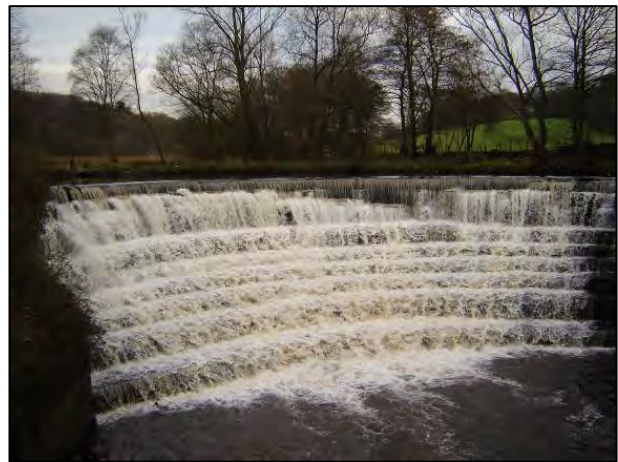
Weir. An impressive curved and stepped structure with a dramatic fall of water, designed to generate power for the mills. Nearby sluices allowed control of the water levels.
