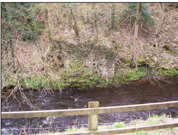
Remains of the trestle bridge abutment that carried the tramway from Ernecroft Wood drift mine to the canal quayside. Evidence remains of both coal workings and the tramway embankment.
