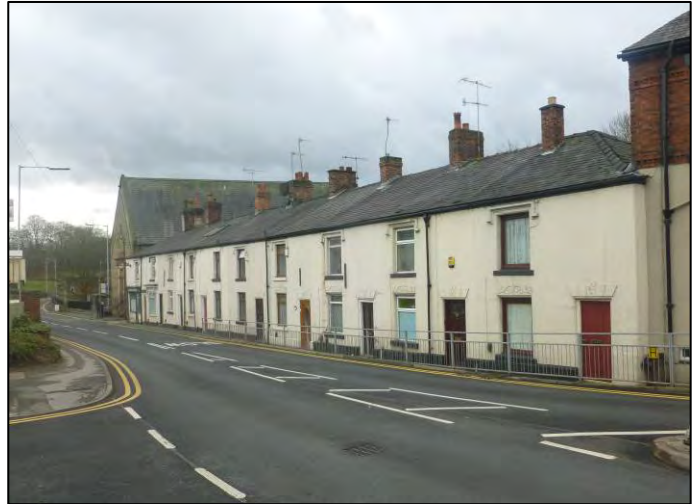
Stone detailing to Andrew Street terraced houses. Upper windows have Tudor-style hood moulds, while ground storey lights have shaped lintels with incised decoration. Door lintels are wedge-shaped and rusticated with incised keystones. These small houses are unusual within the village in being so elaborately decorated.
