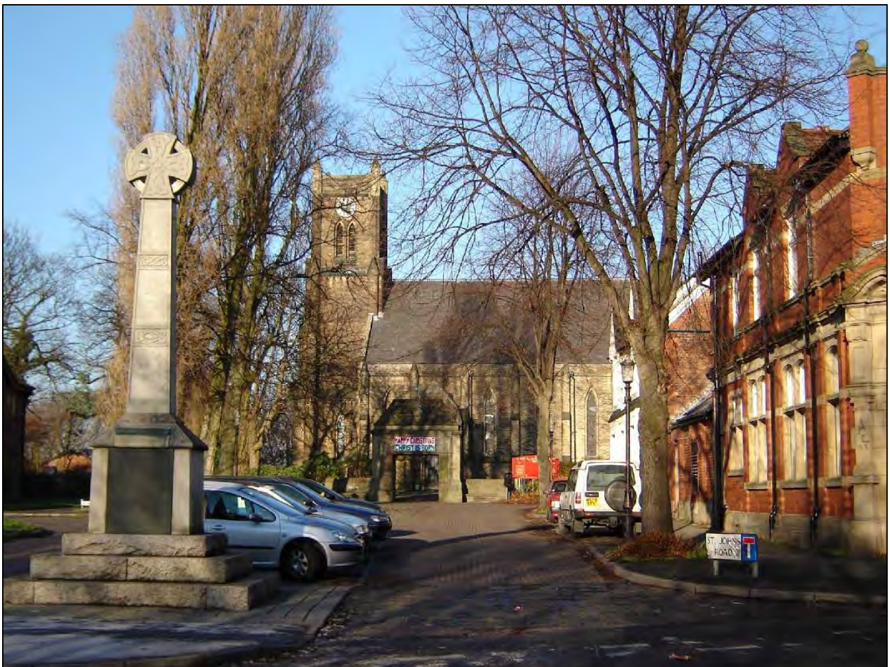
St. John's Church, set on a formal approach along St. John's Road with the axis defined by the war memorial, monumental lych gate and the south porch.
