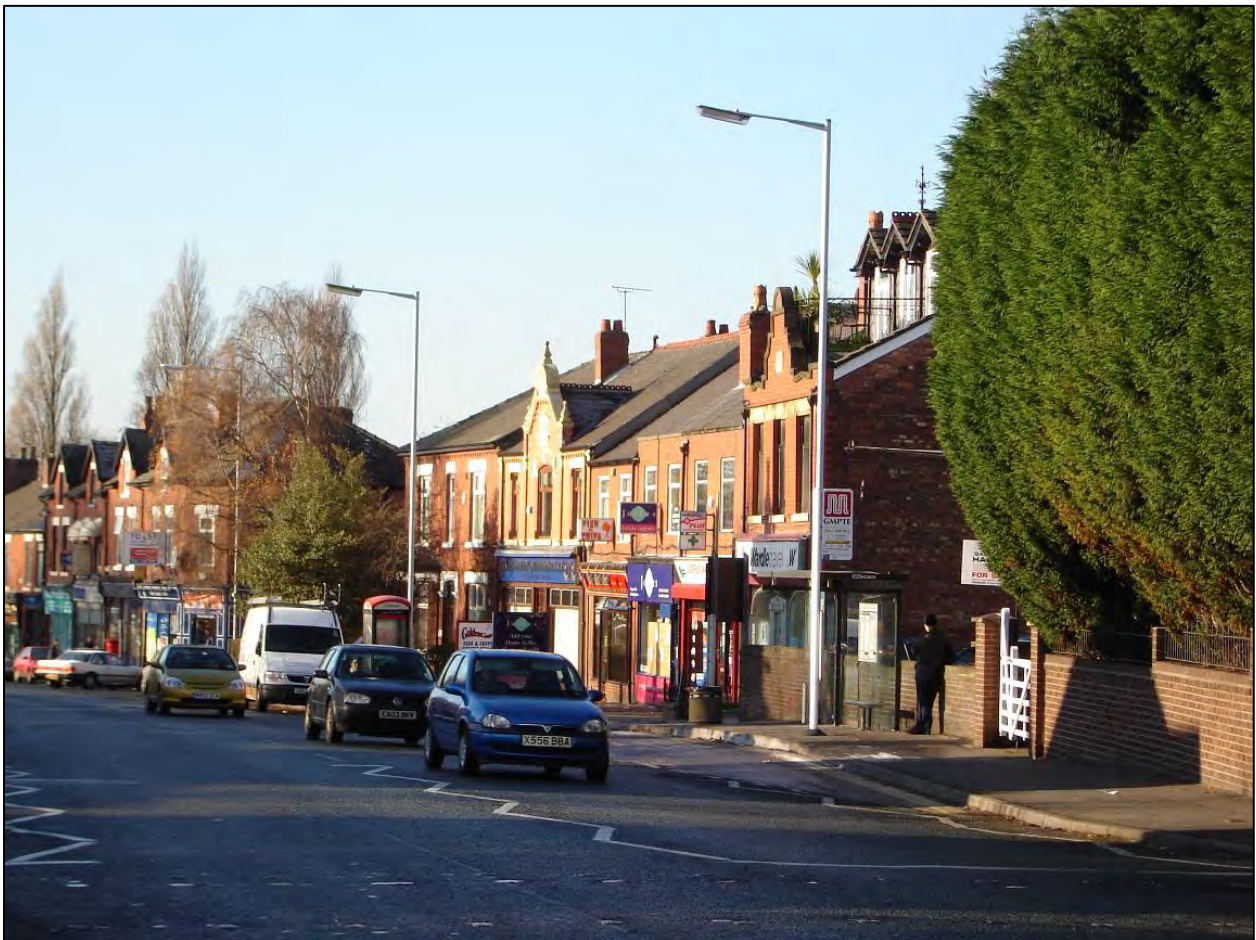
Commercial buildings on Didsbury Road, looking west
