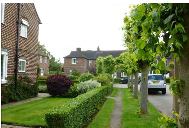
Neo-vernacular cottages and landscaping at Pleachway
