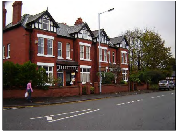
445-451 Didsbury Road , forming with its mirror image and the Richmond Road terraces an architectural set piece on the edge of Heaton Mersey Park
