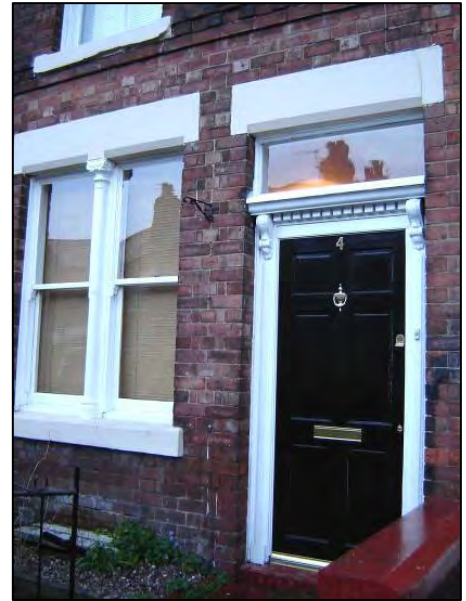
Attractively detailed windows and doors, Lyme Street
