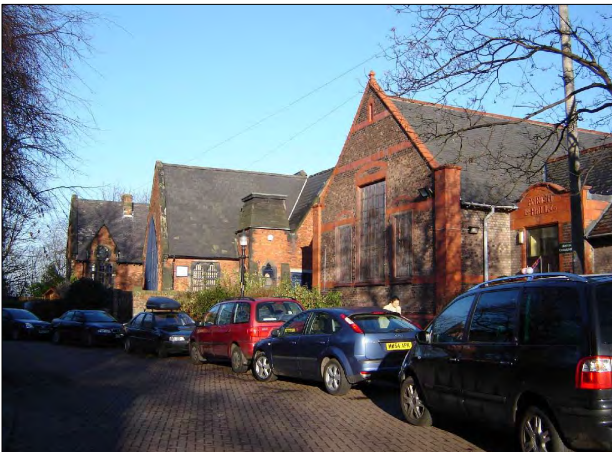
Former St. John's C of E Primary School and the Parish Hall (foreground)
