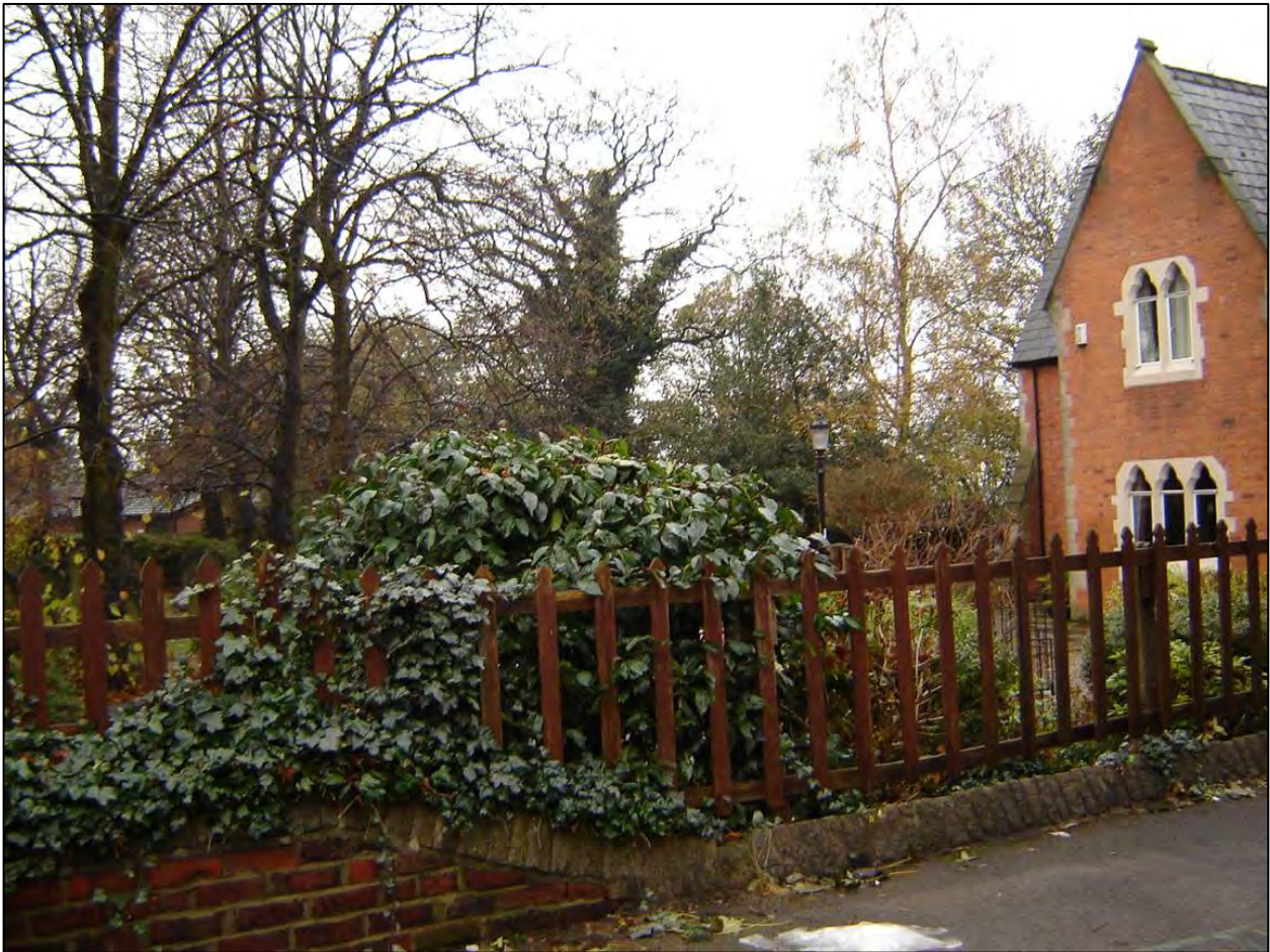
Former Schoolmaster's house, No. 10 St. John's Road
