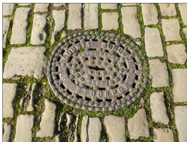
Manhole cover, Vale Close
