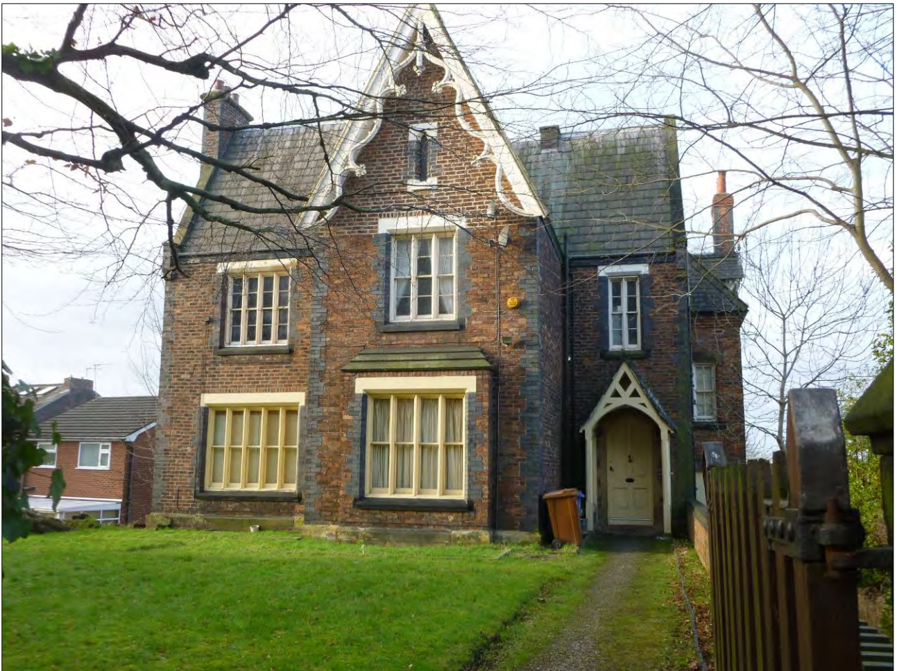
Beechwood, 12 St. John's Road
