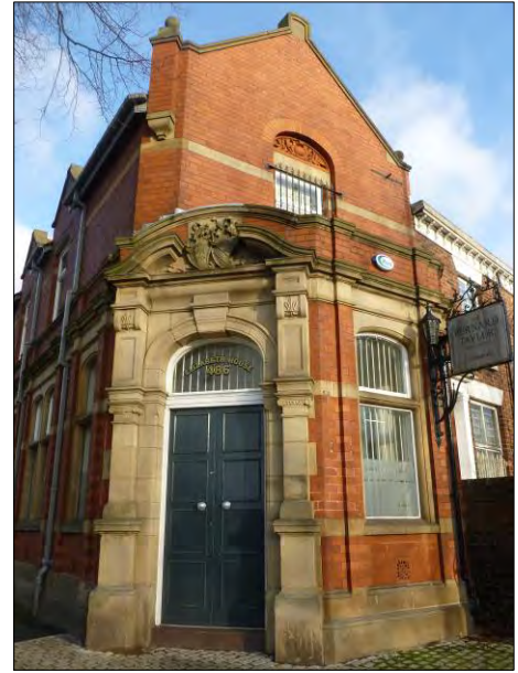
Former bank at the corner of Didsbury Road and St. Johns Road, c. 1900. Glowing local red brick with carved stone dressings: a good local example of the free use of classical detailing in the Edwardian period.
